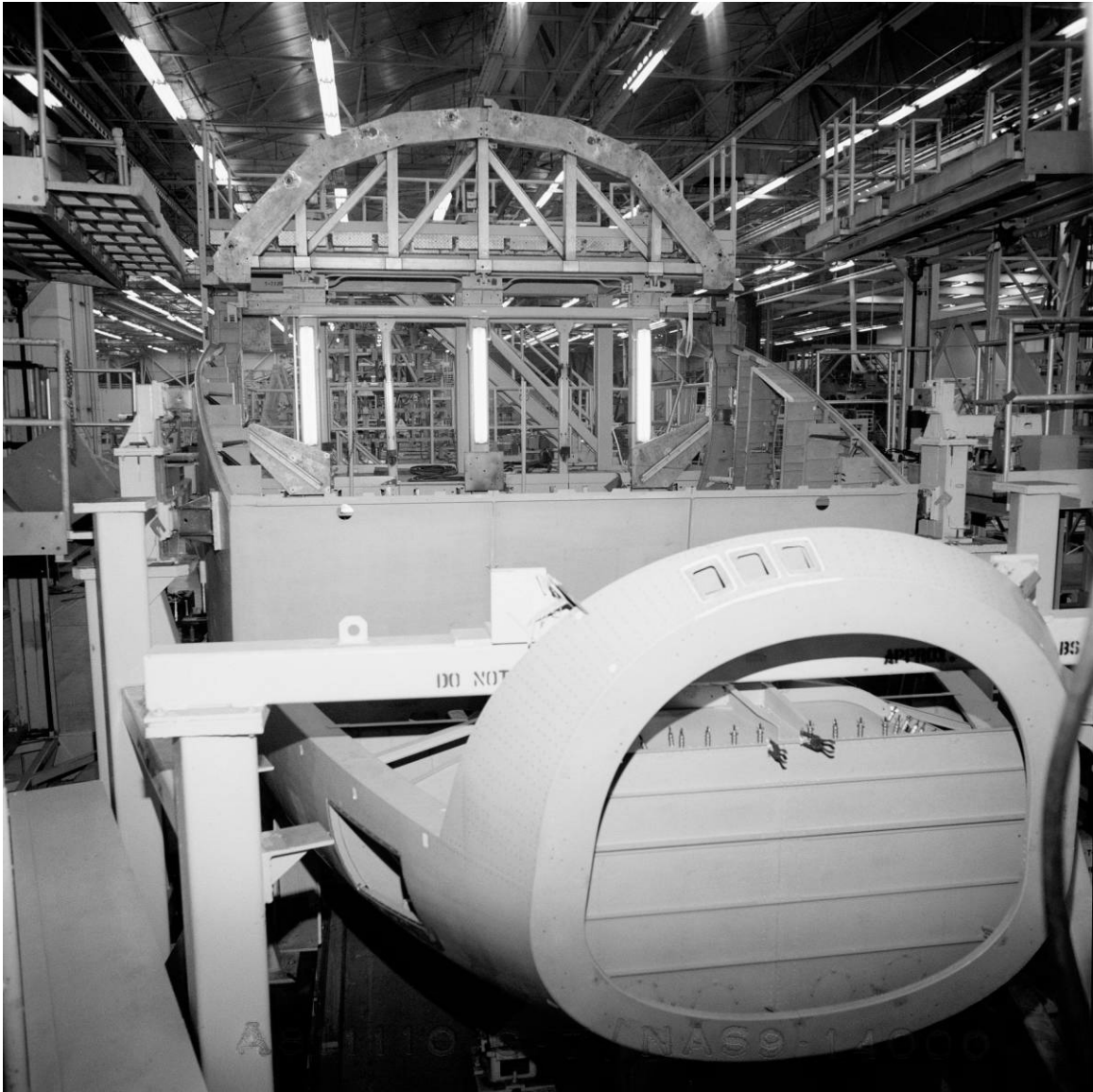
Figure B-2. Manufacturing of Discovery's lower forward fuselage, NAR Building 290, Downey, California, November 10, 1981. Source: NASA, Johnson Space Center Image Repository, JSC2010-03198.
